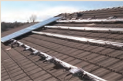
Installation of MicroPV kits on rooftops showing rail-mounted micro-inverters.
