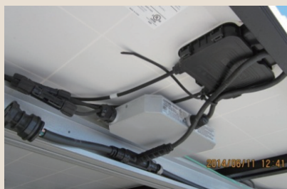
The MicroPV ® system allows a micro-inverter to be mounted on a rail underneath a solar panel.
